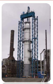
A tower system, 36 metres high, with a single L450 strand jack was prepared to lift the reactor while it was being dressed out. The reactor was moved to the foundation on April 5th, The next day a test lift to 110% of actual weighttook place and the lift commenced immediately thereafter. The lift was completed in 2½ hours.
