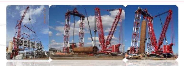
Fagioli was contracted for the on-site transportation and installation of 80 Piperacks and 57 vessels for the Hydrotreaters 2B Project.
